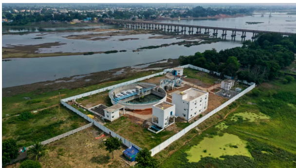
Photo: 7.6 MLD STP on Mahanadi River
