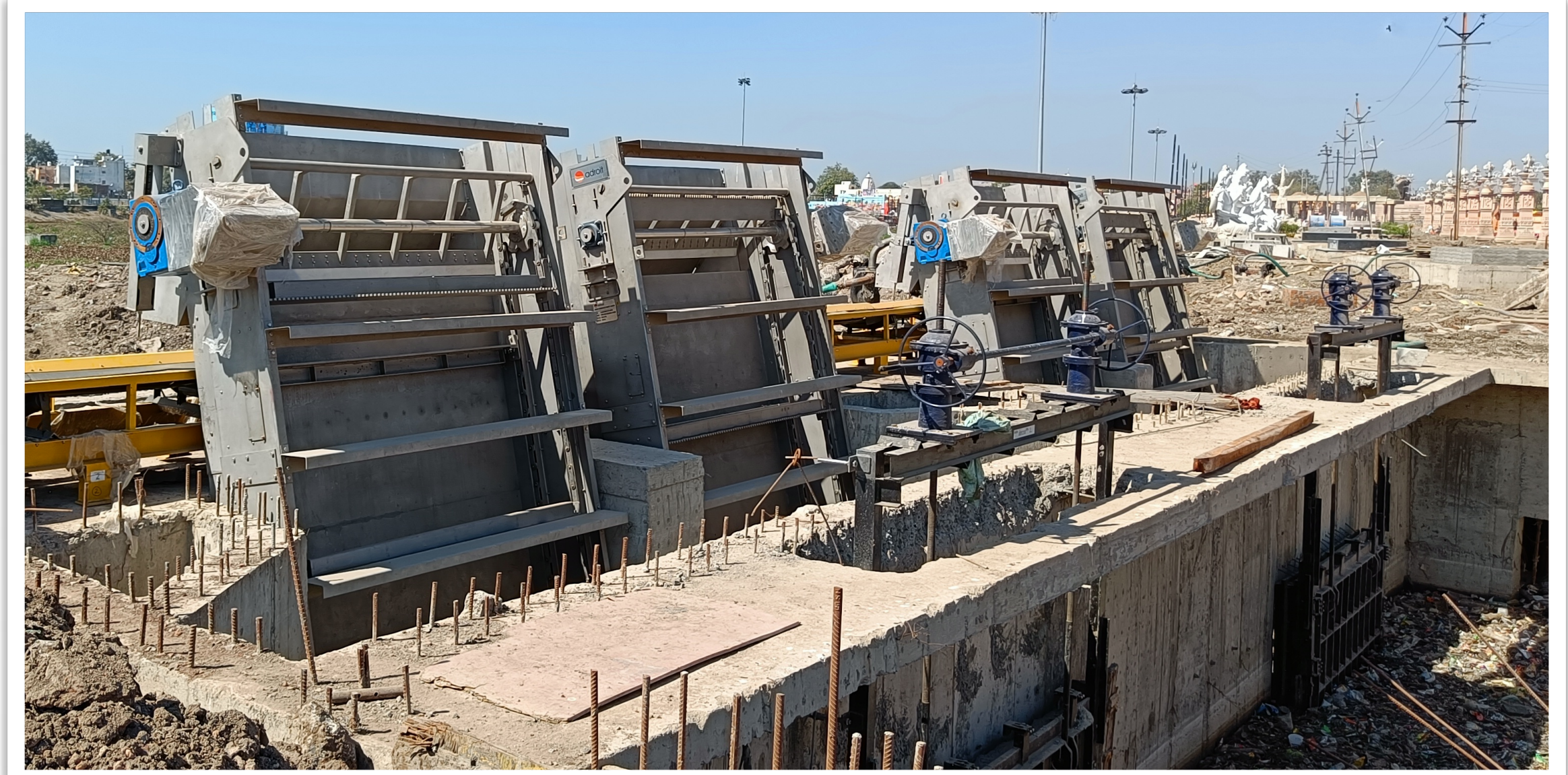
Our installation of 4 Multi-rake Mechanical Screens, 5 Sluice Gates and Conveying System at storm discharge outlet at Rudra Sagar Lake
